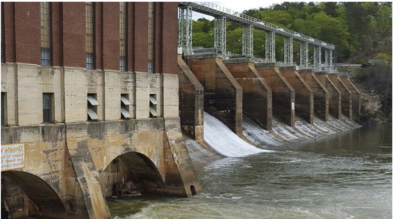
Figure 1 | High Rock hydro power plant.
