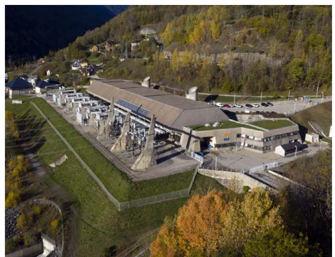
Figure 2 | Aerial photography of Grand Maison PSD switch yard and top of the powerhouse. Photo by: Matthias Magg.
